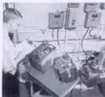
The Type 1554-A Sound and Vibration Analyzer with the Type 761-A Vibration Meter, as set up for the measurements on an air compressor (see Figure 4, page 5).
